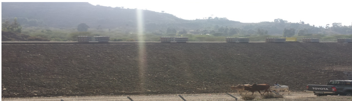
Figure 3: The railway embankment under construction (Feb, 2016)
