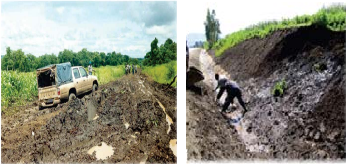
Figure 10: Problems due to expansive soils occurred on the Ethiopian roads [16]
