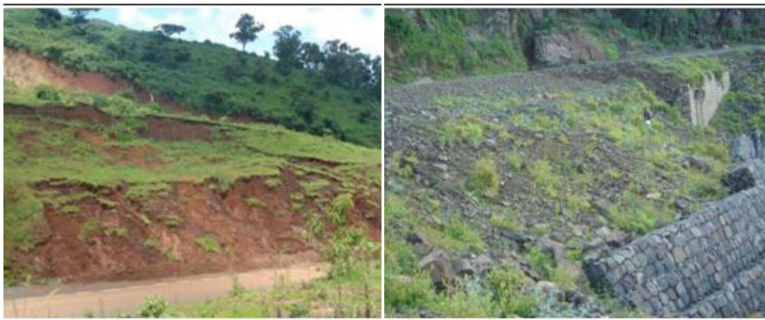
Figure 5: Earthslide affecting an asphalt road in Ethiopia [2]
