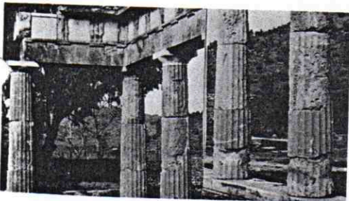
Weathered ancient columns and intercalated recently constructed drums, Stoa, Vravra
